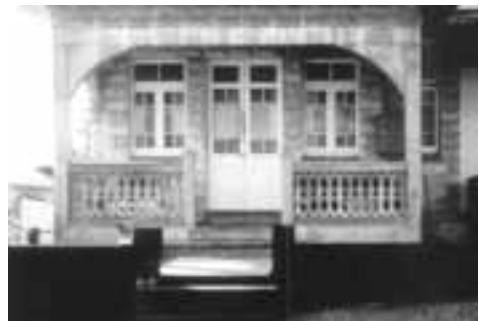
Cement and brick construction was an Italian specialty. This house at 23 Mourilyan Road was built by Emilio Campi circa 1924.
