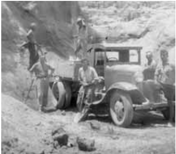
Men digging sand to make a new road through the bush.
